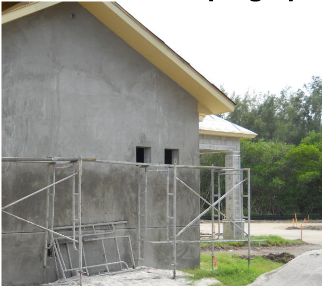
Upper Left- Stucco begins over the styrofoam insulation
