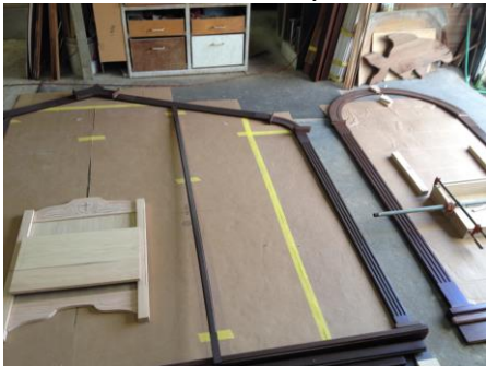
wood Trim for new window ready!
