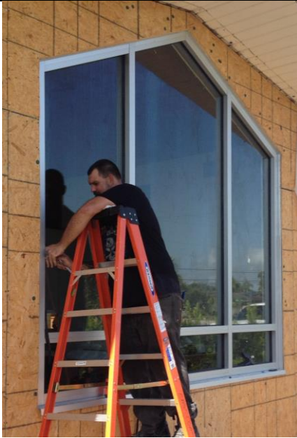
North window finally installed!
